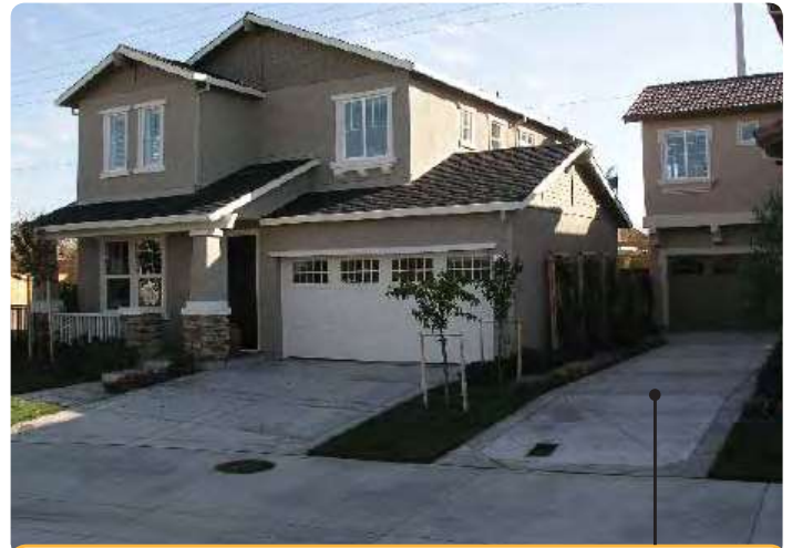
Variation in garage placement, driveway widths, and concrete scoring to create a more engaging streetscape.
